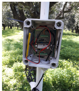
Fig. 3. Installation of the AREThOU5A IoT end-node in a perennial olive field.
