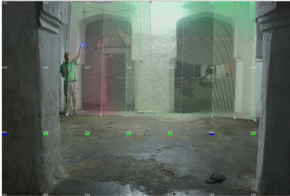
Figure 3 Tippu Tip House base level. Almost no air circulation.
