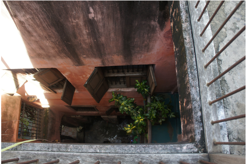
Figure 4 Sokomohogo 478 open shaft with a plant growing at the base level.
